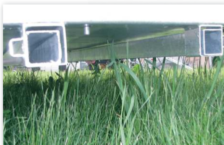
Square tube beams
